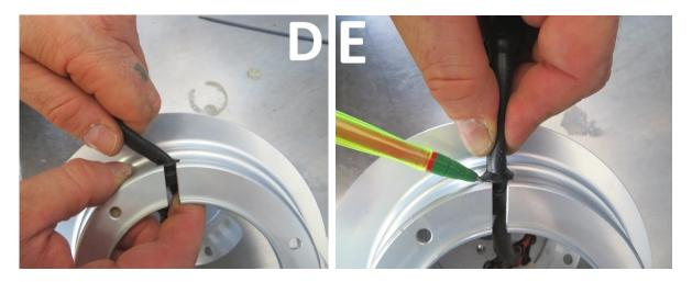
Now gently pull the sleeving through the main hole, doing so from one side, and then the other (see **Pic. D**), until the lip of the cast-in grommet of the actual sleeving pops through the hole, as can be seen in **Pics. E** + **F.** Using a little silicon spray will assist greatly in doing this.
